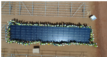
Installation of solar panels at Essakane. Image courtesy of IAMGOLD.
